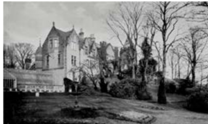
Cowden Castle, showing the probable 1893 additions (forward) and surviving turret (to the right).
